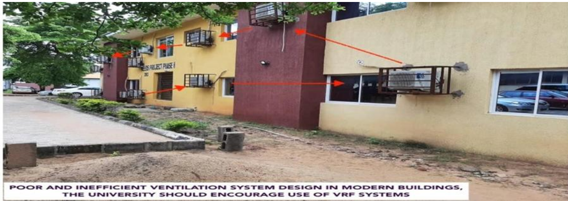
Figure 12. Poor and Inefficient Ventilation System Design
